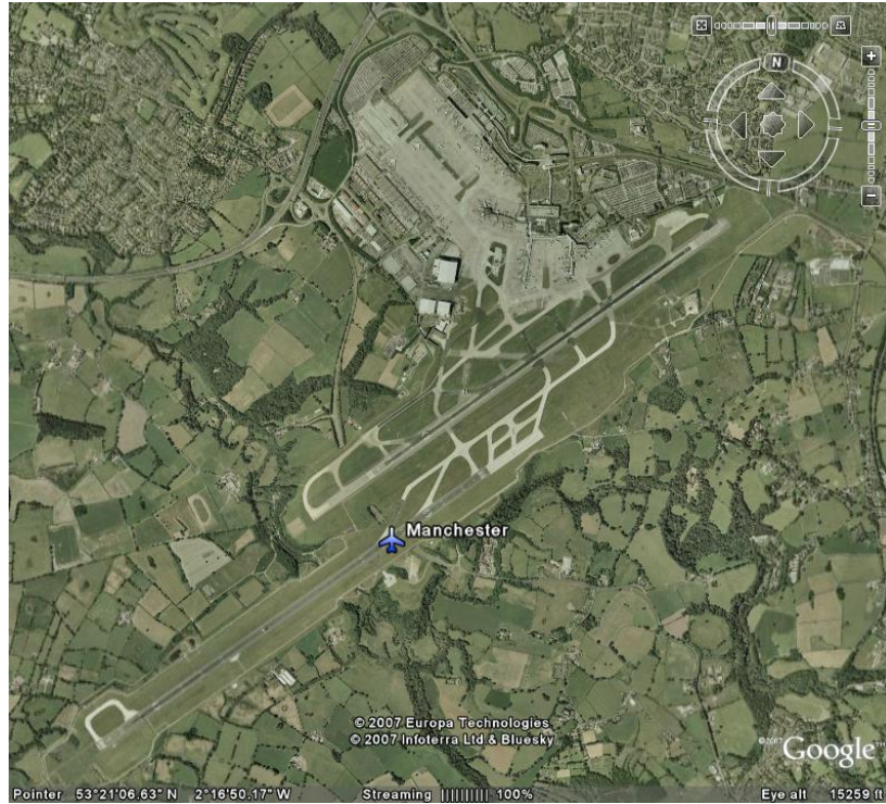
Fig 5.6 Manchester International Airport, although a wide-spaced runway is more preferred on enhancing capacity, land take is always a major obstacle for airport development worldwide that would limit the choices available [Photo courtesy of Google Earth 2007]
